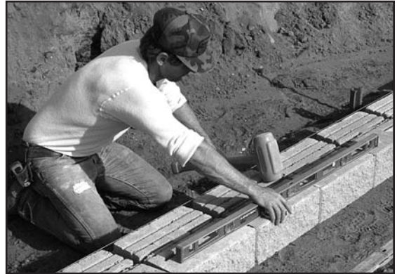
7. Use a long level to maintain consistency unit to unit.
