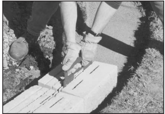
6. Use a VERSA-Lifter® to aid in lifting and placing base course units.
