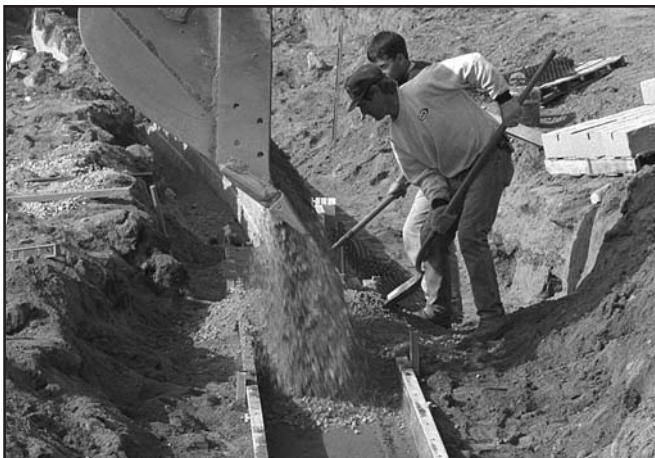
3. Fill forms with granular base material.
