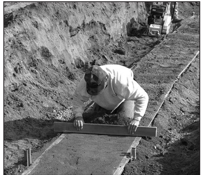
5. Screed sand for final leveling of pad.
