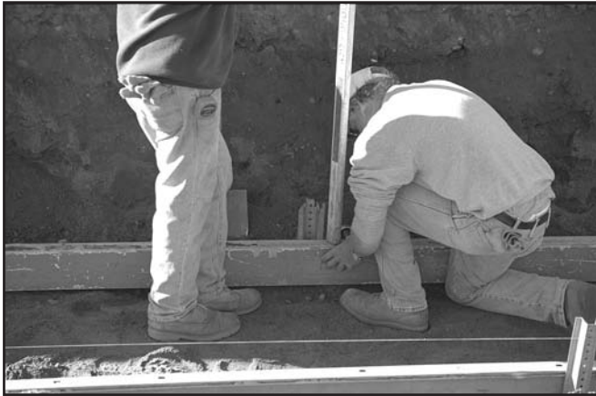
1. Set and level metal screed forms.
