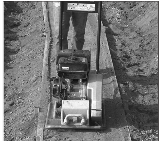
4. Compact leveling pad granular material.
